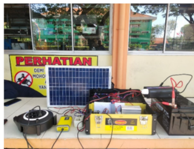
Figure 4. On-grid based IoT PLTS circuit
